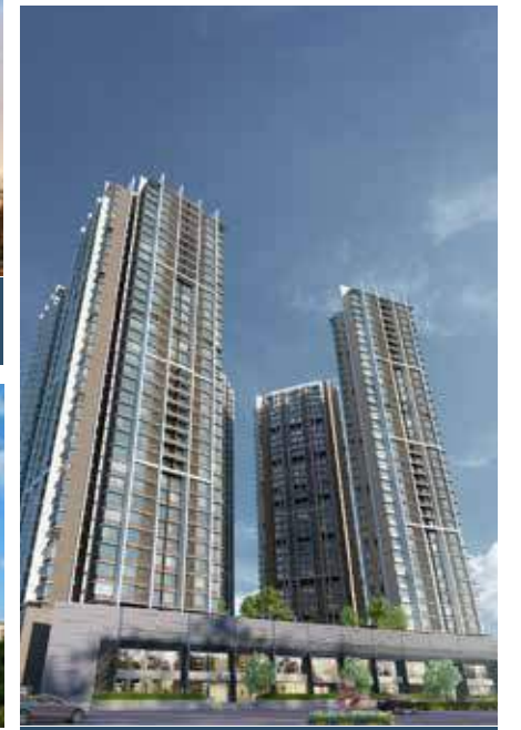
Kalpataru Paramount Thane (W)
