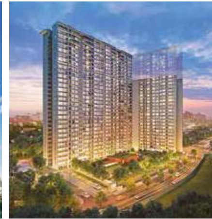
Kalpataru Magnus Off BKC
